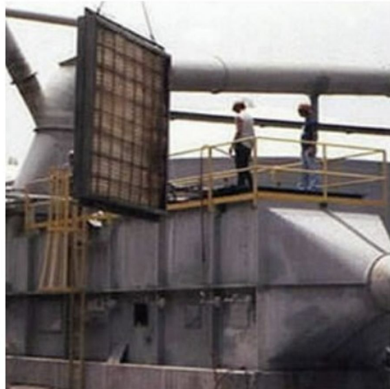
Kimre tower packing, mist eliminators, cassette frames and supports are installed in the user's vessel. Kimre provides design support for new vessel construction or retrofit of existing vessels, and offers new vessels or "packaged" systems.
