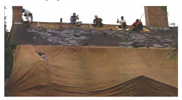
If the leak is coming from damage to the roof deck, you'll need to remove shingles to gain access to the damaged section.
