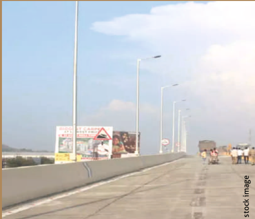
8 Lane Highway (Work in Progress)
